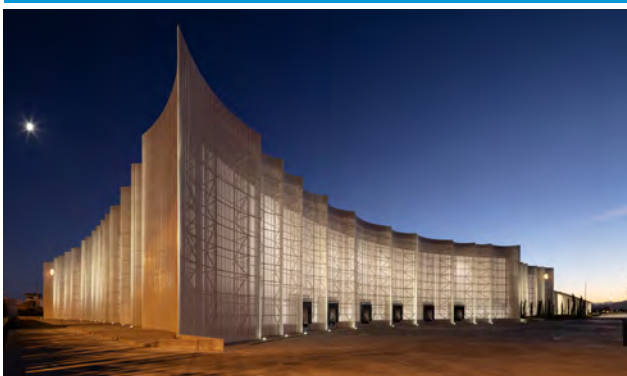
Total Clima Málaga - Logistic Center
